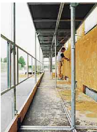
Decking consists of an aluminium frame with anti-slip protected plywood.
