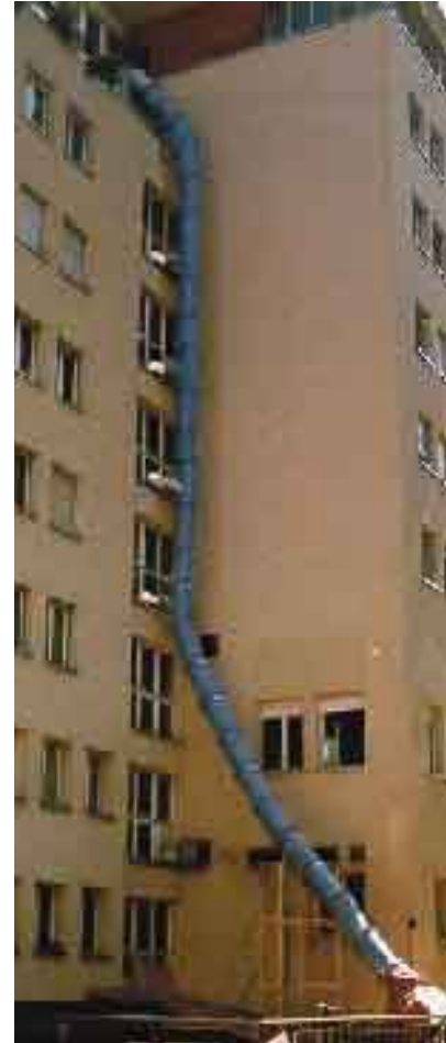
Our rubbish chutes are corrugated on the inside for increased rigidity and endurance.
