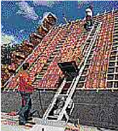
A lift on an inclined slope will save time and prevent injury when for instance putting tiles on a roof.
