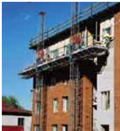
Using double masts the platform can be up to 30 m wide.
